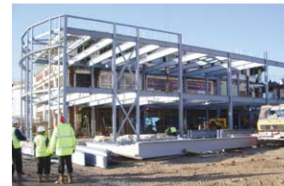
The new conference suite on the north wing taking shape - Nov 06
