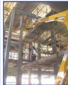
New vent Shaft & staircase (left) – Recent steel erection of the vent shaft core in the Royal Hall.
