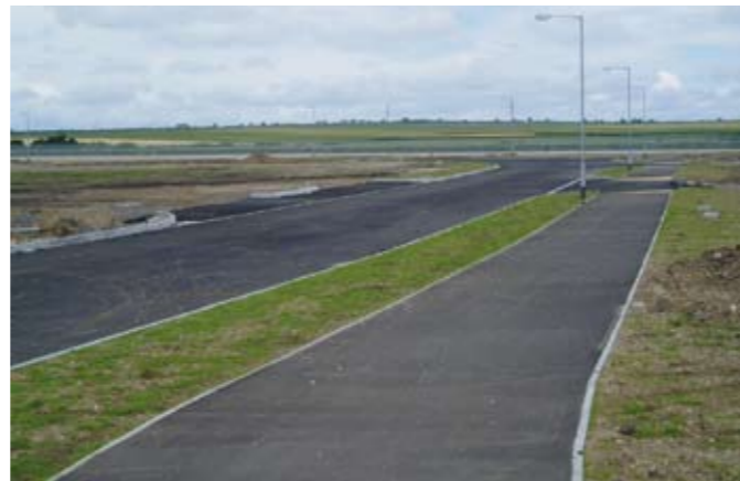
AFTER: The site off Lancaster Road at the beginning of July
