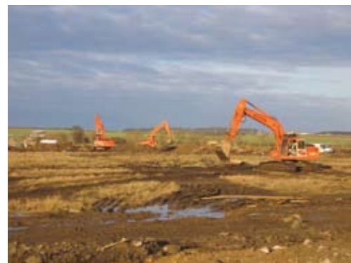
BEFORE: As the JCBs started work at Carnaby
