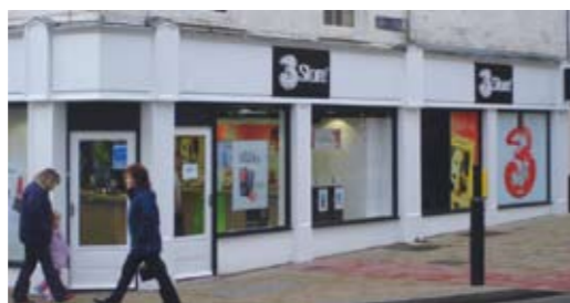
3 Store - Chapel Street
