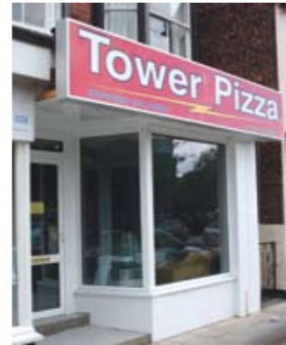
Tower Pizza, Quay Road
