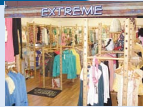
Extreme Clothing, Chapel Street. Internal refurbishment
