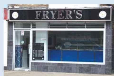
Refurbishment - Fryer's Fish Shop, Flamborough Rd.
